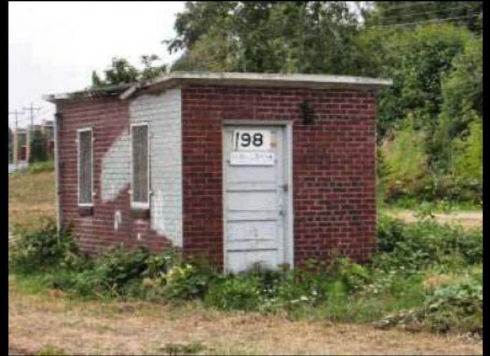
Gasoline Pump House
