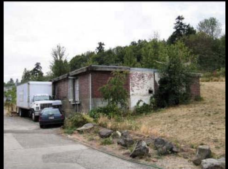
Tank Farm Repair Shop
